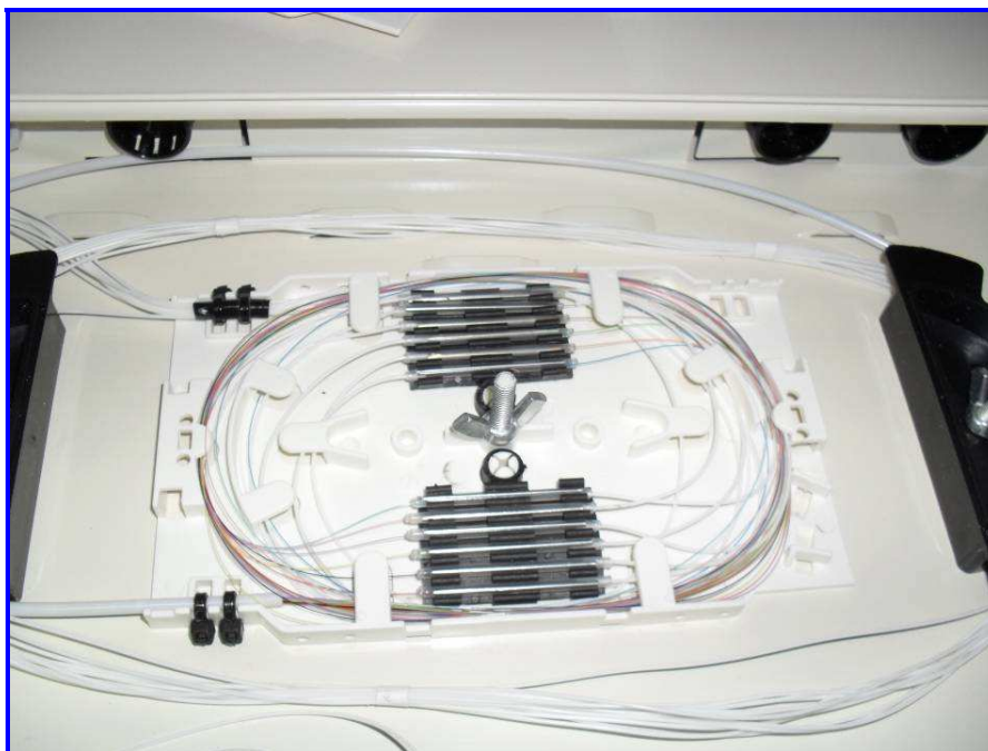
Figura 11. Fusiones patch panel PAO
