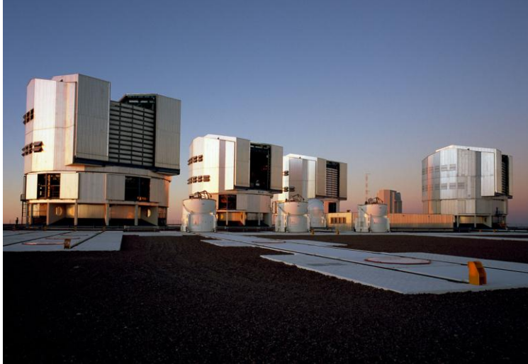
Figure 1. The Very Large Telescope (VLT) on Cerro Paranal. Each enclosure hosts an 8.2m telescope. Note also the four smaller enclosures in the foreground, each hosting one of the four 1.8m movable auxiliary telescopes used for interferometry.
