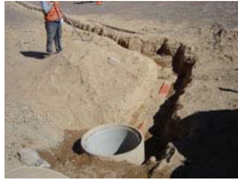
Figure 7. (Right) excavation for the installation of a concrete manhole (left) that will host the splicing box used to connect two consecutive sections of cable, about every 4km.
