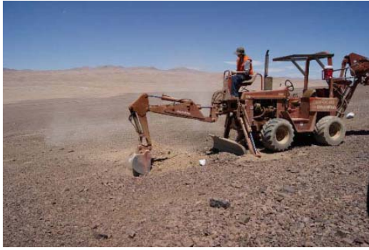
Figure 7. (Right) excavation for the installation of a concrete manhole (left) that will host the splicing box used to connect two consecutive sections of cable, about every 4km.
