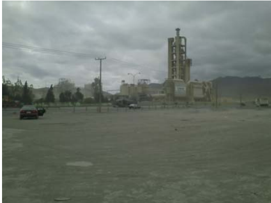
Industrial complex in La Negra
